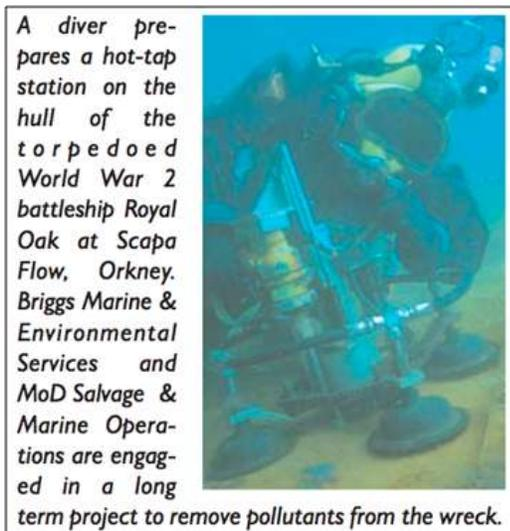
Figure 3.4 – Diver hot tap similar to techniques adapted for ROV use (ASA).
