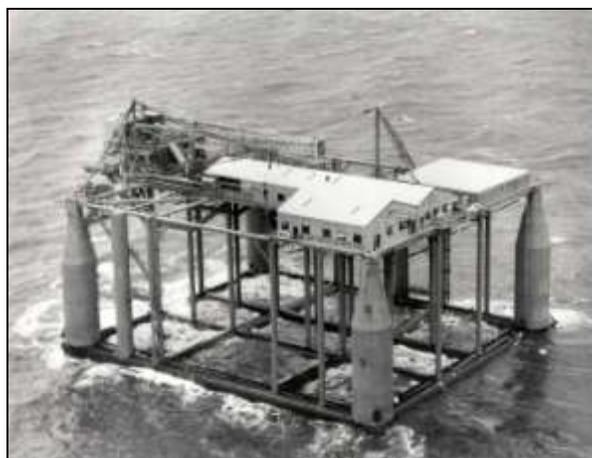
**Figure 4.1 – Photo of Bluewater Rig No. 1, the world's first semisubmersible drilling vessel.**<sup>15</sup>
